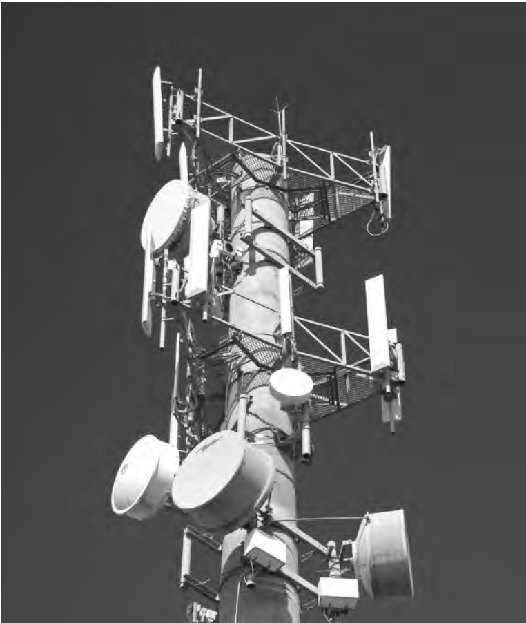
FIGURE 3.12 A microwave tower. The round antennas are microwave antennas and the straight antennas are cell phone antennas. Source: Matej, Pribelsky listock photo
